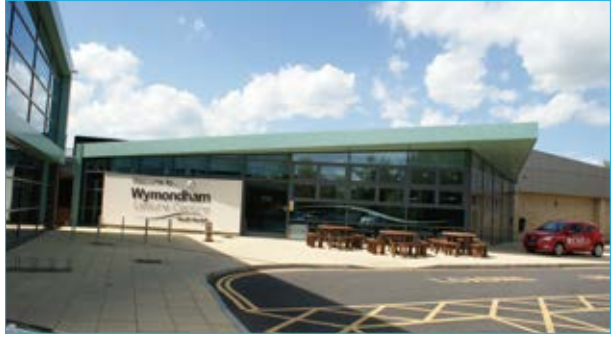
Wymondham Leisure Centre GMV5 Heat Recovery UK
