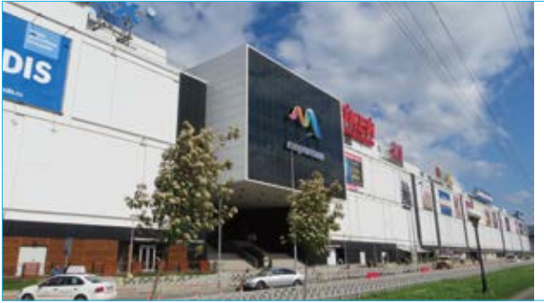
Sochi More-Mall Centrifugal Chiller Russia
